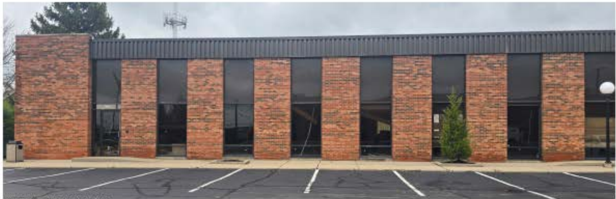
EXISTING CONDITIONS PHOTO
